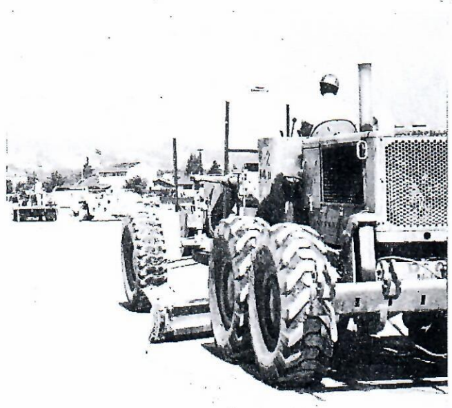
GRADER operator watches the target and adjusts blade to keep the laser beam between reference marks.
