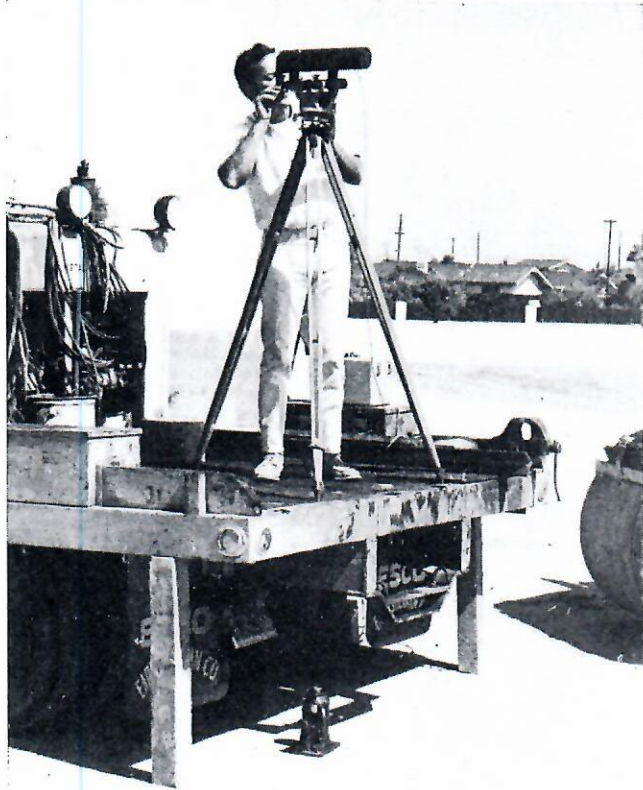
POSTS under truck bed stabilize it to provide a solid platform for the laser. Power supply is truck battery.
