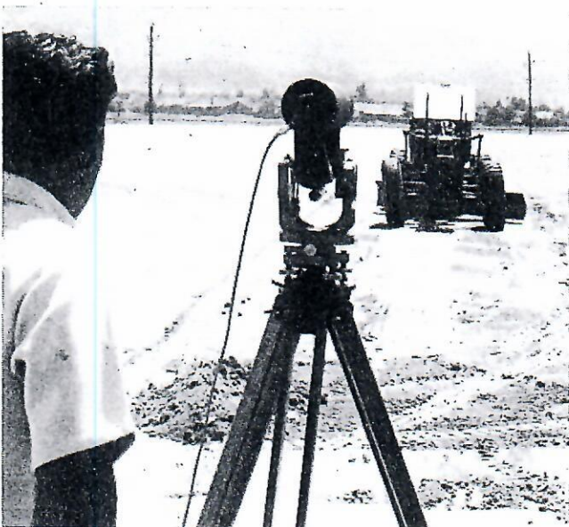
LASER beam projected through transit optics provides elevation reference for grader blade.
